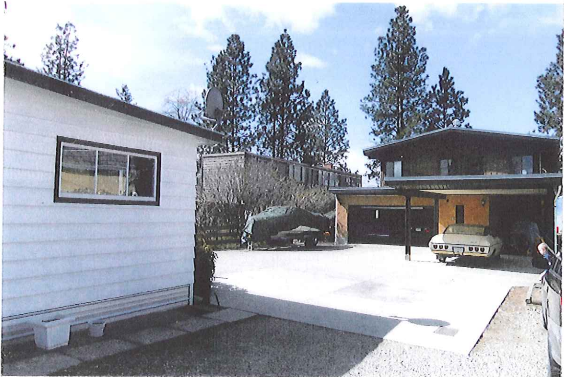
VIEW OF DISTANCE BETWEEN COTTAGE + HOUSE
